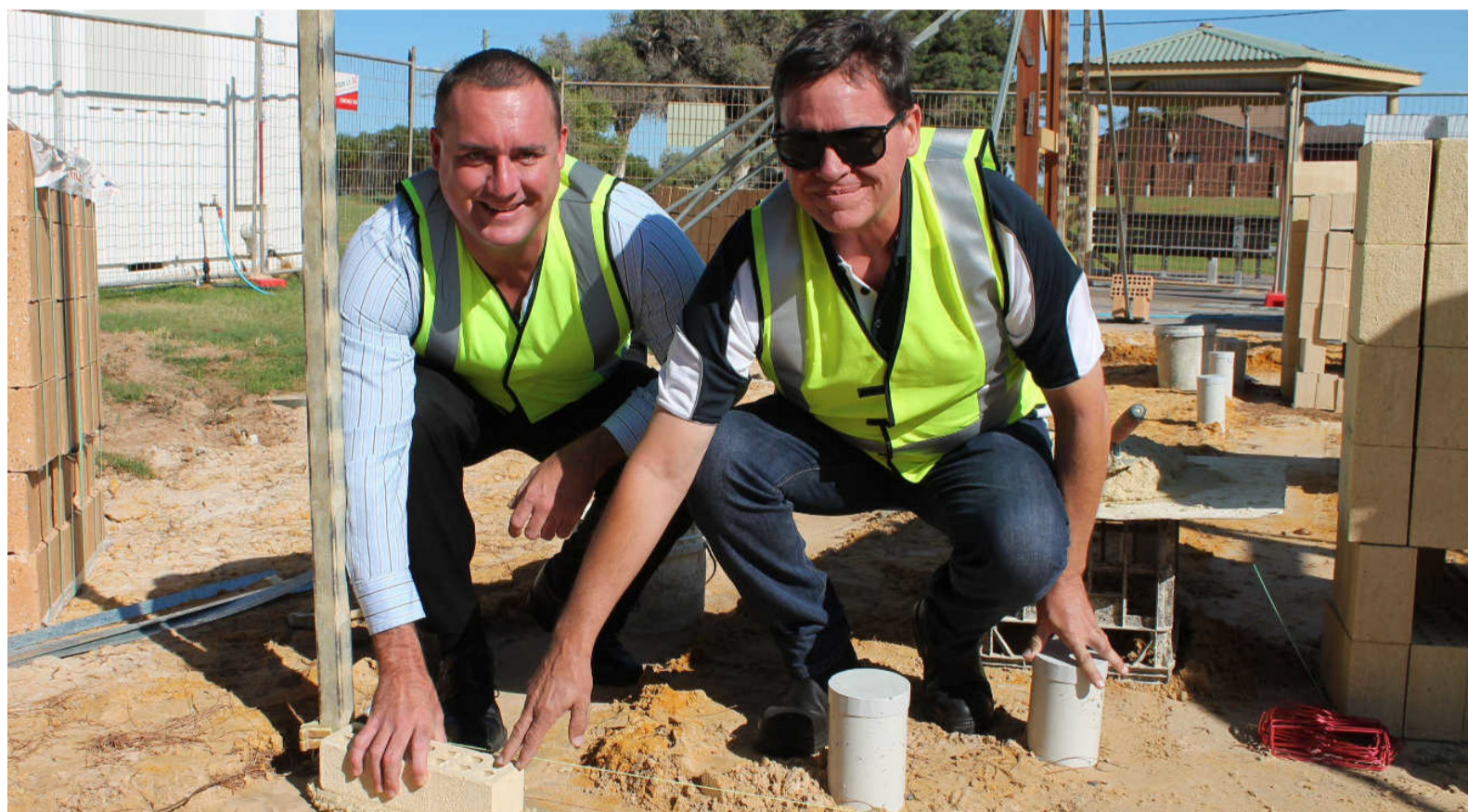
City of Greater Geraldton mayor Shane Van Styn and WA Country Builders Mid West general manager Phil Raven lay the first brick of the new toilets.
